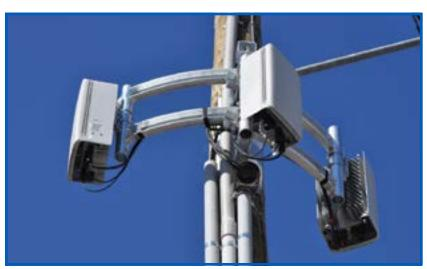
97-5GWDMTHGN1-A installation with (3) customer-supplied 5G radios
