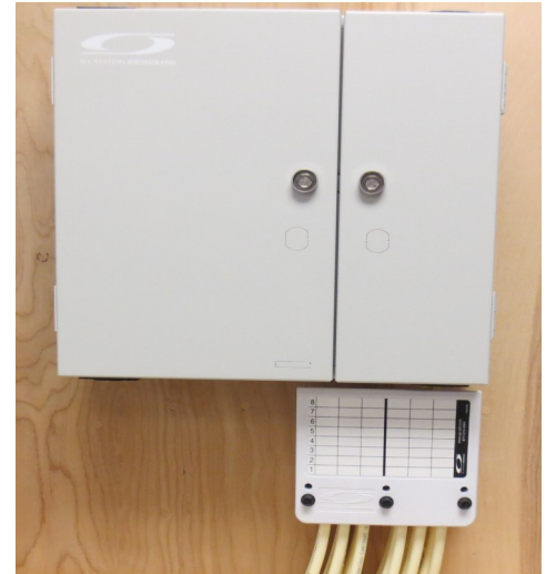
Microduct Manifold with Enclosure
